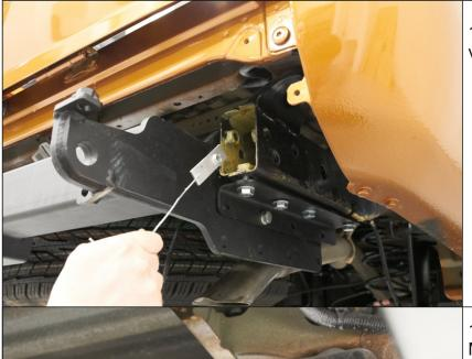
11. Mount inside nut M10 (I) into the vehicle frame from the right side.
